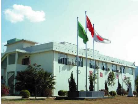
Office and Refrigerator-House
